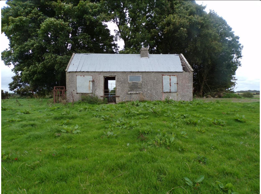
Plate 14-5: Vernacular building CH46, facing north.
