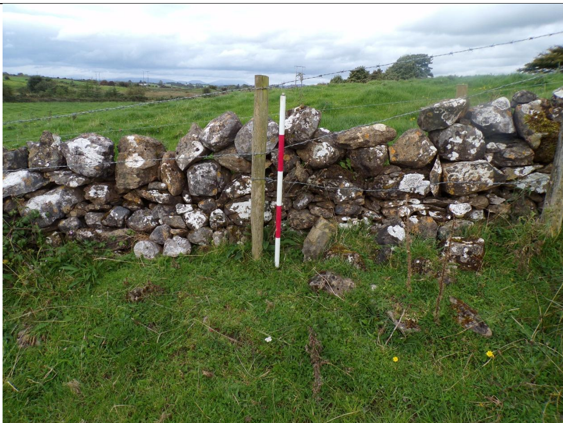
Plate 14-10: Drystone wall at location of substation, facing north.
